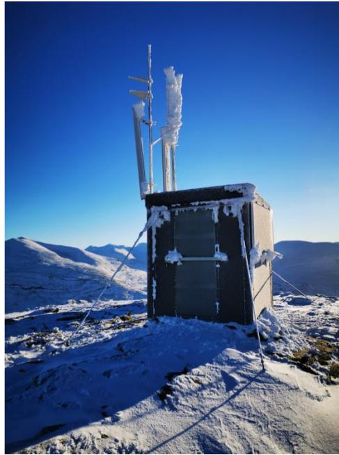
Figure 48 A rural hot-spot giving 2G and 4G coverage. Power comes from solar panels and fuel cells. Edge computing could be installed here. Photo: Mats Jonsson, the #fulltäckning project.
