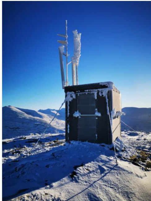
Figure 19 A rural hot-spot giving 2G and 4G coverage. Power comes from solar panels and fuel cells. Edge computing could be installed here. Photo: Mats Jonsson, the #fulltäckning project.
